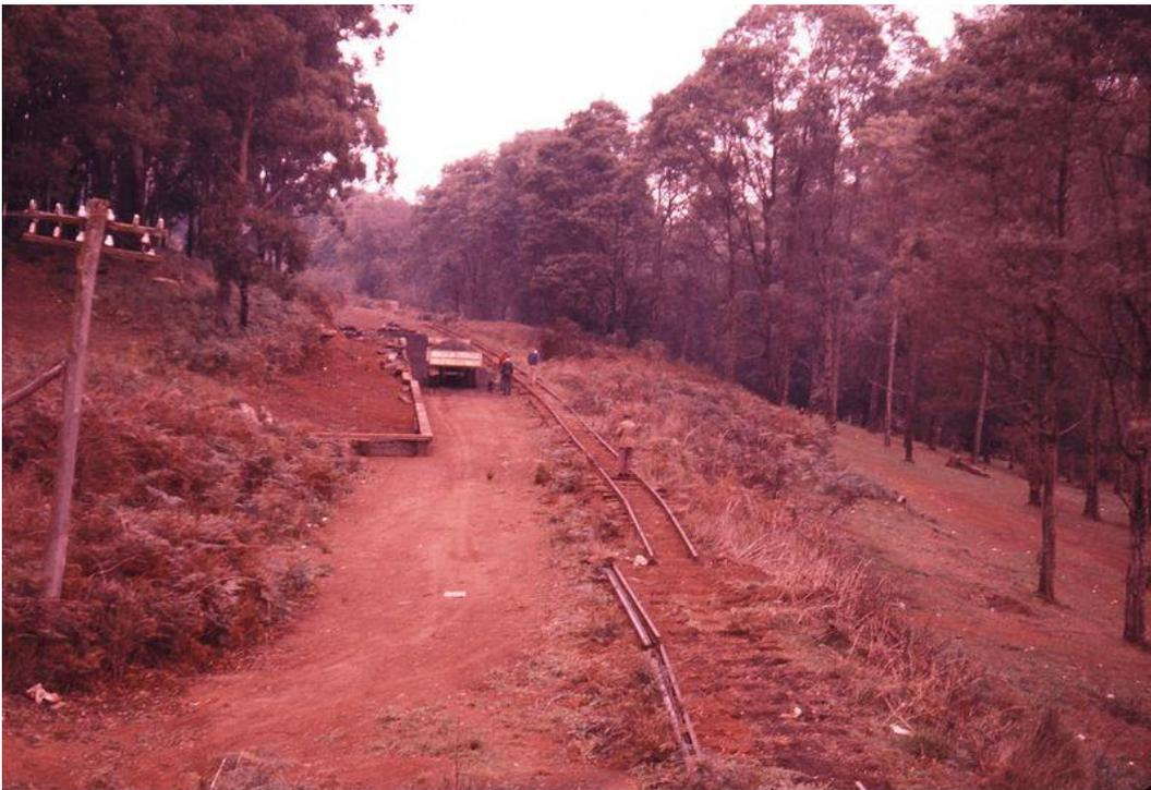
**Plate 28 Lakeside Station platform construction and re-laying of ballast by the PBPS in 1961 (Langford, 2004)**
